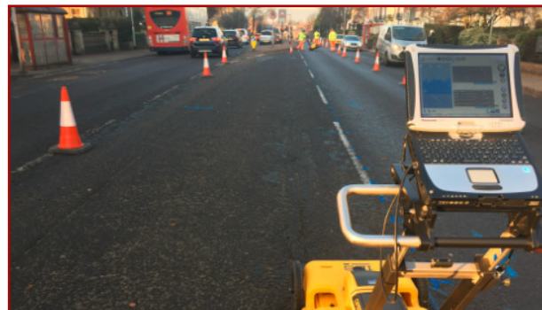
Underground Utilities Survey
