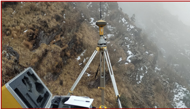
Establishment of Control Point
