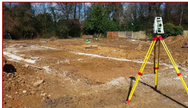
Setting Out Survey
